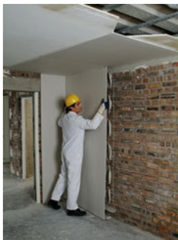
Figure 4 – Application of internal insulation
