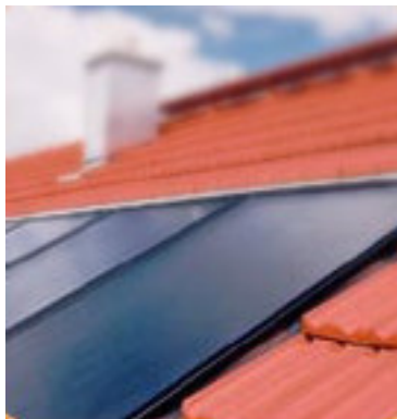
Figure 14 – Active solar thermal panels
